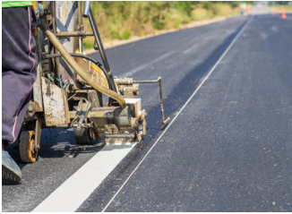
Enhanced Pavement Markings
