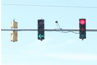
Left-turn Signal Phases (Protected and Protected-Permissive)
