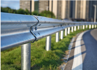
Guide Rail Upgrades
