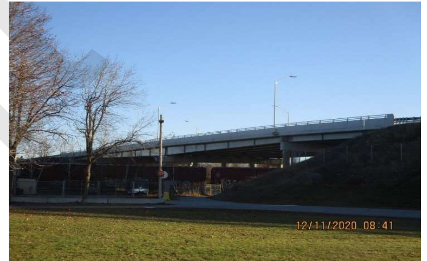
Very Good Condition – Lakeshore Overpass
