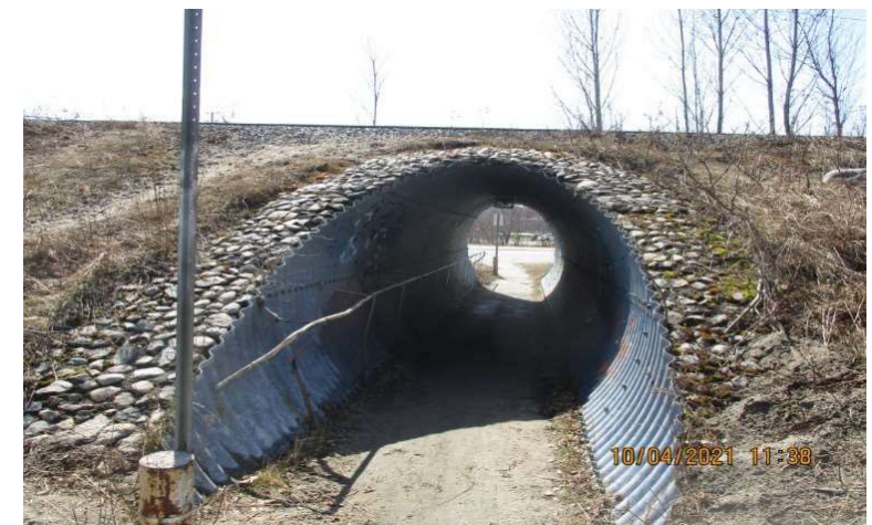
Ski Club Road – ONR Underpass – Fair Condition Culvert
