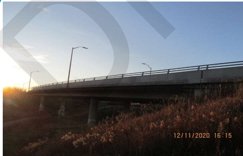
Trout Lake Overpass – Fair Condition
